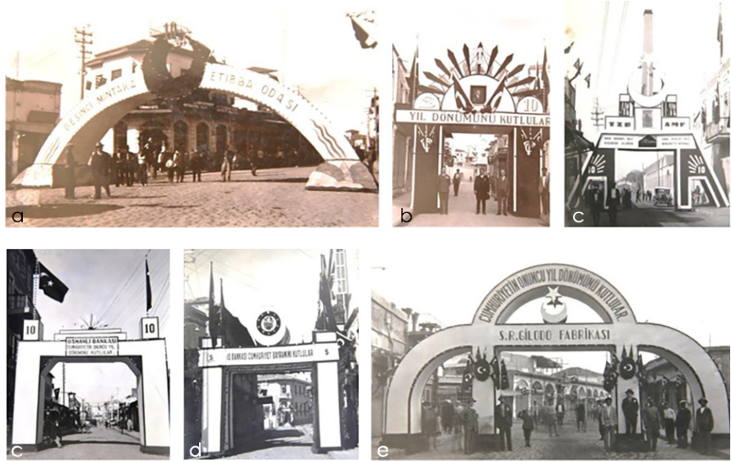
Figure 5. a) Tak of the Chamber of Physicians, b) Tak of Ziraat Bank, c) Tak of Salonika Bank, d) Tak of Ottoman Bank, e) Tak of Is Bank, f) Tak of S.R. Gileto Factory (Kalafat & Kalafat, 2022)- Adana, 1933.
