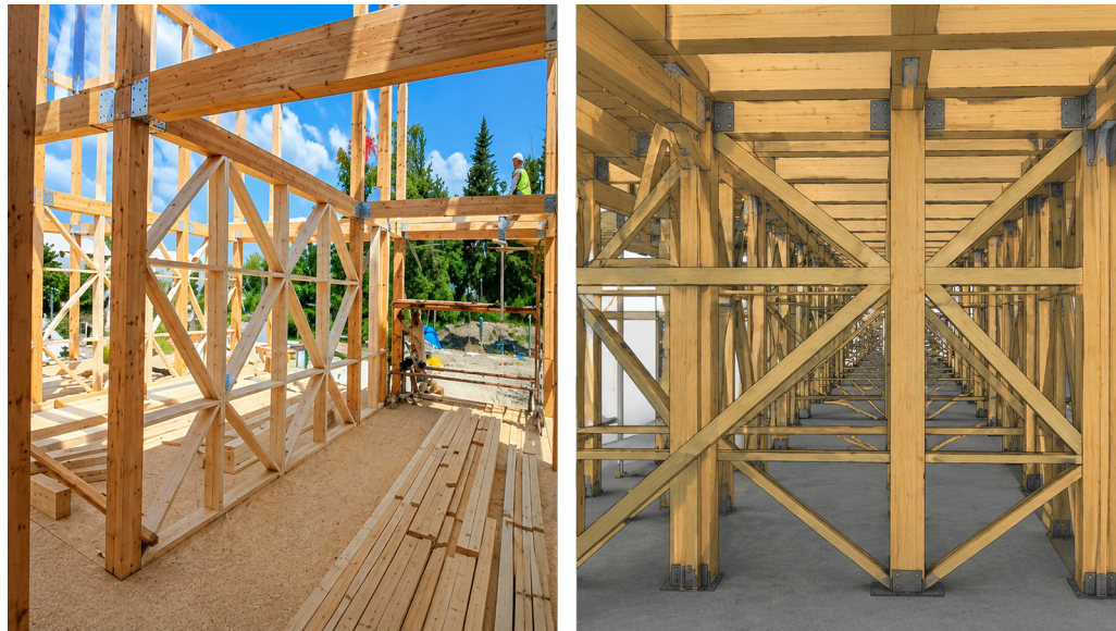
Figure 4. Wall frame of the Osmaniye Timber Housing Project (Unpublished company working report, 2023, NASWOOD).
